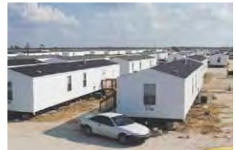
FEMA mobile homes being set up in Port Charlotte, Florida, to provide temporary housing for victims of Hurricane Charley (August 2004). Nearly a year after the storm, these trailers were still being used. (Photo courtesy of FEMA)
