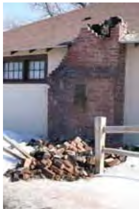
Typical results of moderate earthquake shaking in Idaho: foundations fail and brick chimneys topple. (IGS and NBMG photos).
