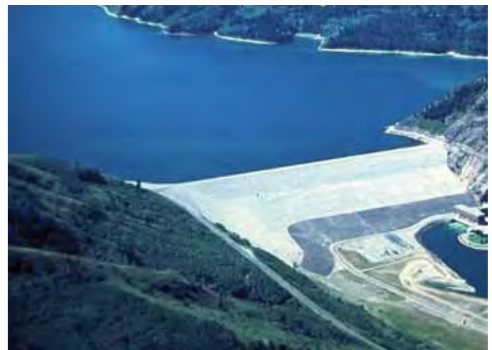
View of the Palisades Dam and Reservoir. Constructed in 1957, the Palisades Dam is 240 feet high and 2100 feet long. It dams the South Fork of the Snake River 18 miles west of the Idaho-Wyoming border. The reservoir is operated to supply about 670,000 acres of irrigated land in southern Idaho, generate about 177,000 kilowatts of hydroelectric power, and control floods. The trace of the Grand Valley fault zone is about 2.5 miles northeast of the dam (Bonneville Power Administration photo).
