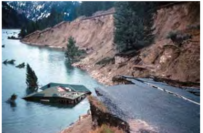
The largest historical earthquake in the Intermountain Seismic Belt was the August 1959 magnitude 7.3 Hebgen Lake earthquake in Montana. Landslides triggered by the shaking submerged Highway 287 (USGS photo).
