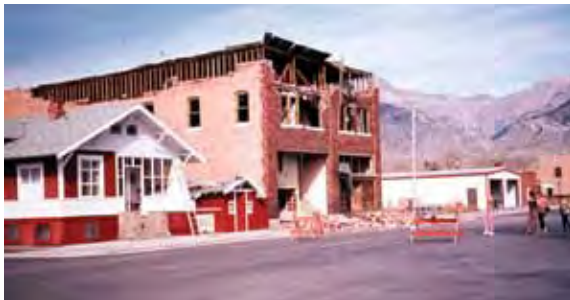
Earthquake damage to the Custer Hotel in Mackay, Idaho caused by the 1983 M 6.9 Borah Peak earthquake. (IGS photo)
