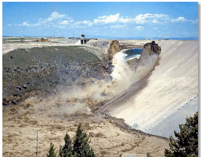
Figure 3.2.R. Teton Dam Failure, June 1976. / Source: http://www.damsafety.org .
