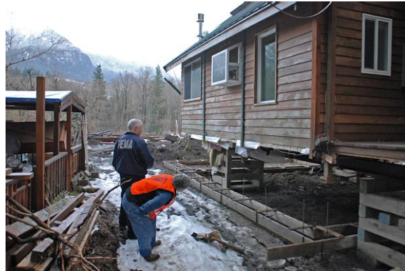
Two men looking at a home being elevated
