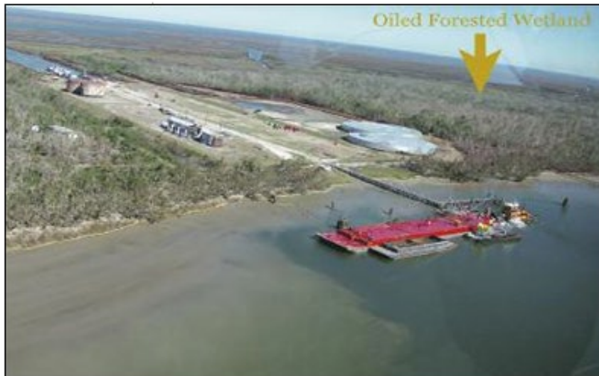
Figure 2: Oil from damaged tanks was moved by hurricane forces into impassable forested wetlands. USCG photo.
