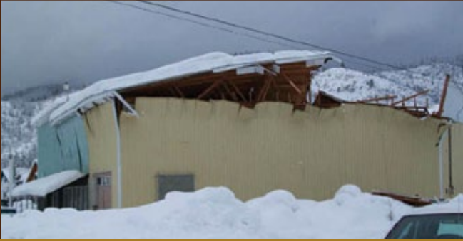
In 2008 in Shoshone County, severe snow loading collapsed roofs, causing damage to homes, businesses, and government buildings.
