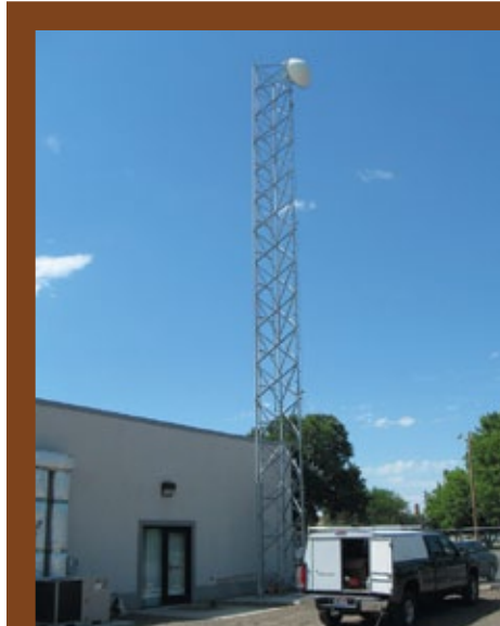
Gooding County Broadband Connection. Gooding, Idaho
