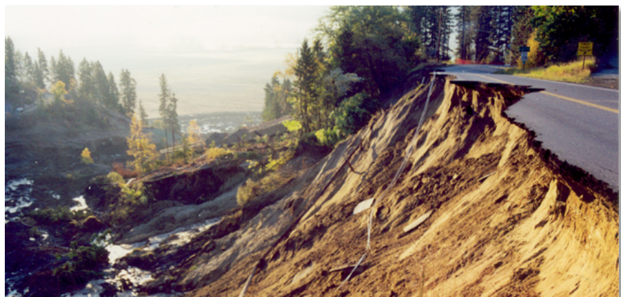
Figure 3.7.C. Earth Flow Damage to U.S. Highway 95 near Bonners Ferry
