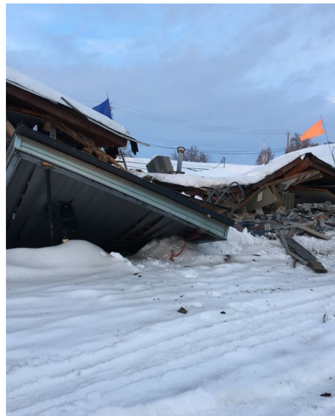
January 2017 Bowling alley in Weiser (Washington Co.) buckles under the weight of snow on the roof; such roof collapses caused widespread destruction
