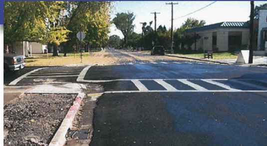
After Mitigation - After .24" of rainfall
