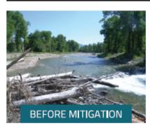
**Problem:** Teton Creek, east of Driggs, Idaho, was channelized, which caused banks to fail, the channel to widen, and riparian trees to fall. Tens of thousands of cubic yards of sediment were deposited often in the form of gravel bars that displaced the creek and caused destabilization. Teton Creek threatened millions of dollars in damages to public and private property.
