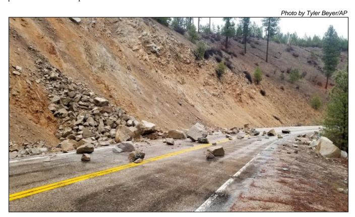
Figure 9-1. Magnitude 6.5 Earthquake Caused a Rockslide on Highway 21 Near Lowman on March 31, 2020
