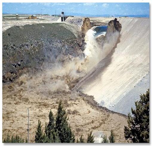
Figure 3.15.F. Teton Dam Failure, June 1976
