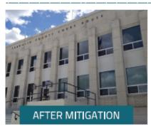
Solution: Historical looking thermal aluminum frames and window panes with bomb blast film replaced the outside windows of the Courthouse to mitigate potential falling glass during an earthquake or windstorm protecting pedestrians below.
